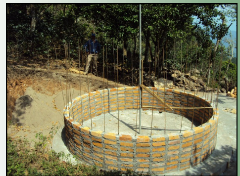
Beginning stages of water storage tank in the community of Zompoperos
