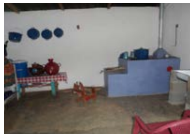
Well-kept kitchens, with plastered and painted walls. / Cocinas ordenadas y con paredes revocadas.
